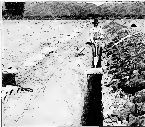
FIG. 81. Construction of a ditch for tile drains.
